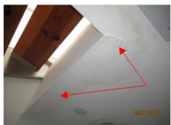
Figure 5: Water damage under stair landing.
